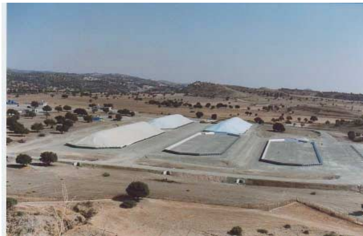
Photo 1: A group of Bunkers of total 70 thousand tons capacity for hermetic storage of grain in Cyprus. An aeration system, controlled by a computer using data from a meteorological station, is installed in two of these Bunkers, to control the grain temperature and moisture migration, to increase the acceptable initial grain moisture content and to remove the phosphine residues after fumigation.
